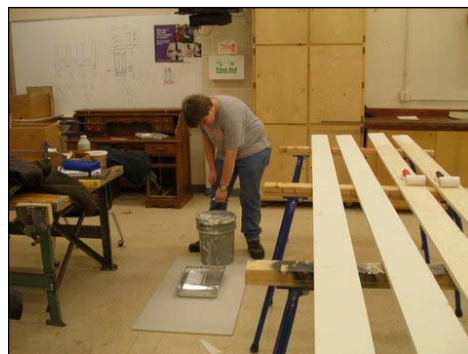
Junior Watson helps prepare the walls for assembly.
