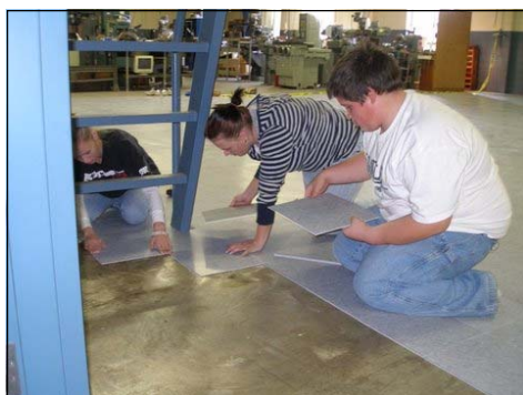
Dorothy Andrews, Danyell Riggins, and Matt Cook lay tile in the new science lab.
